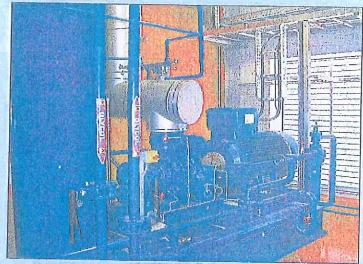
The cascade plant supplies cooling to three cold storage areas and seven blast freezers. Star's refrigeration system is one of the first in Northern Ireland to use CO<sub>2</sub> technology for blast freezing. The Granville plant has a total refrigeration capacity of 1,227kW. The system was designed with sufficient in-built compressor capacity to allow future expansion.
